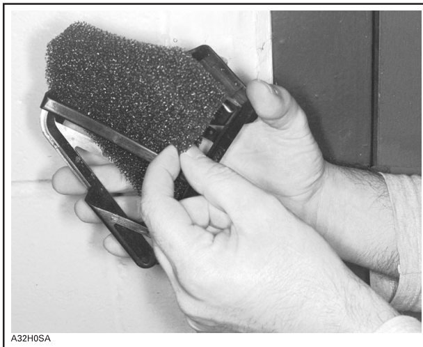
Removal of filter from its grill
