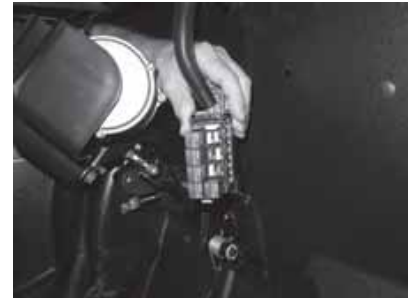
Step 3 - Cover removed
