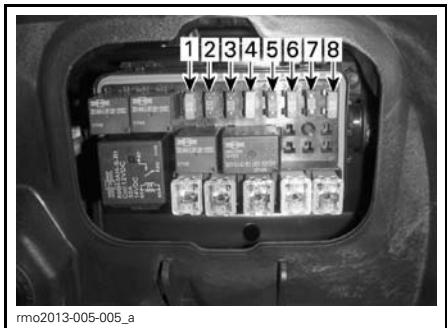
FUSES - LEFT FUSE BOX
