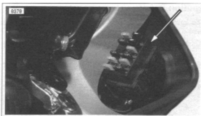
Figure 7-18. Fuse Block (contains diodes)
