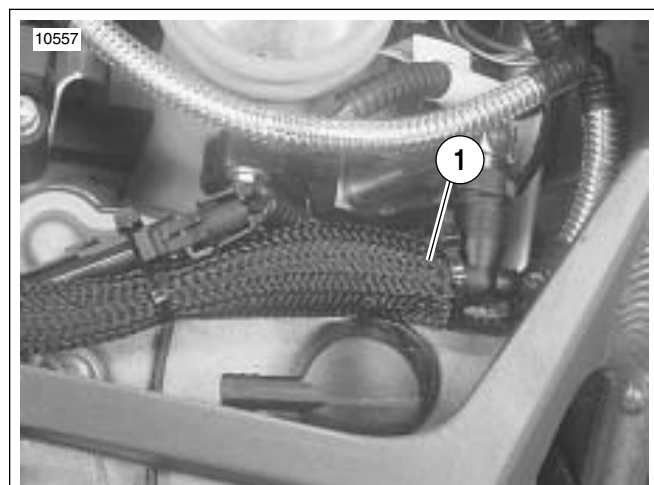
1. Engine temperature sensor connector [90] (approximate location)
